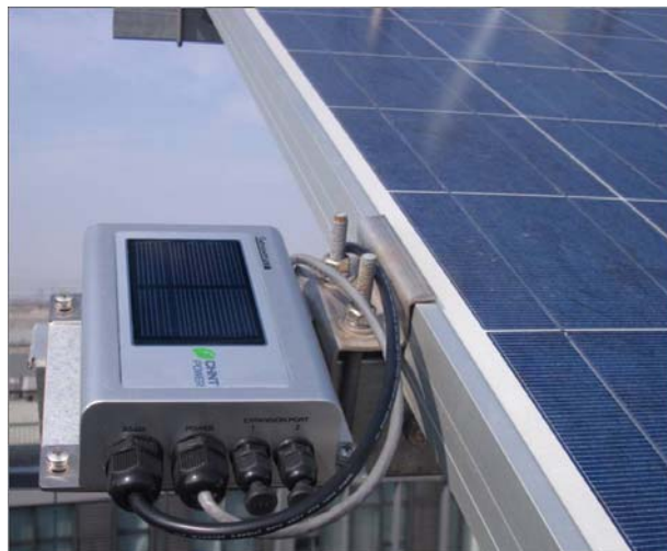
Fig 3-13 Mounting intersensor BOX on PV panel bracket
